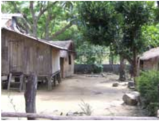
Local Tribal Housing
